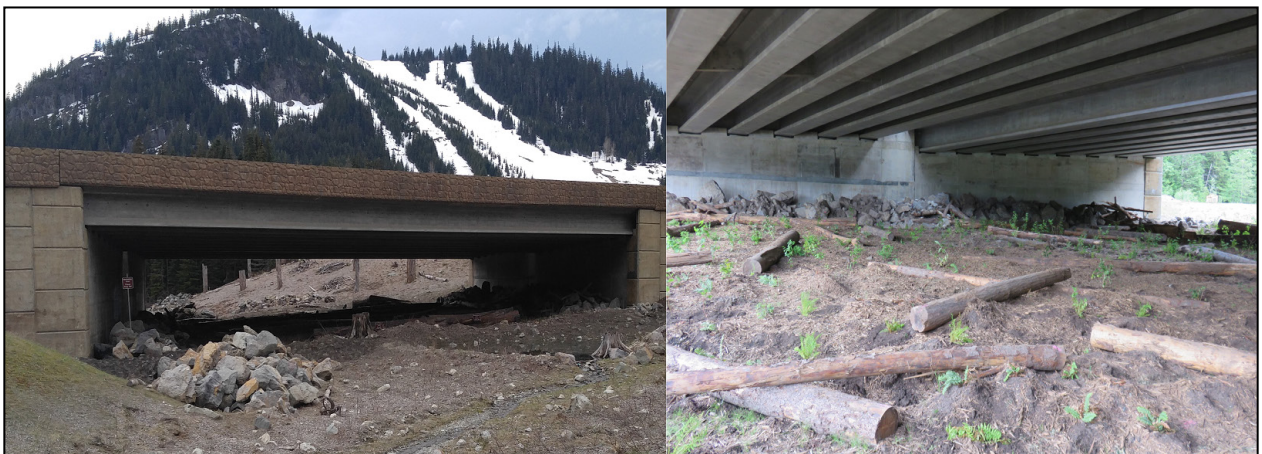
FIGURE 2. The Hyak wildlife undercrossing located at the Snoqualmie Pass in Washington State is an entirely terrestrial crossing structure with native plants, a wood-mulch floor, different sized fallen logs distributed throughout, and rock piles lining the western and eastern borders. (Photographed by Lindsay Millward).
